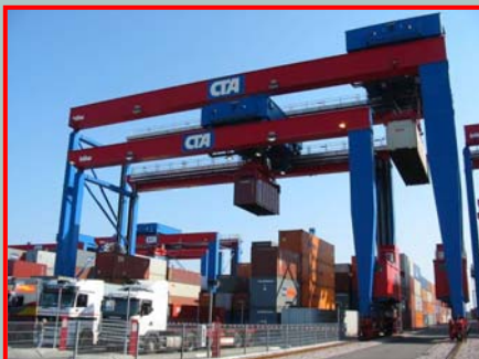
Container Terminal Altenwerder, Hamburg, Germany
